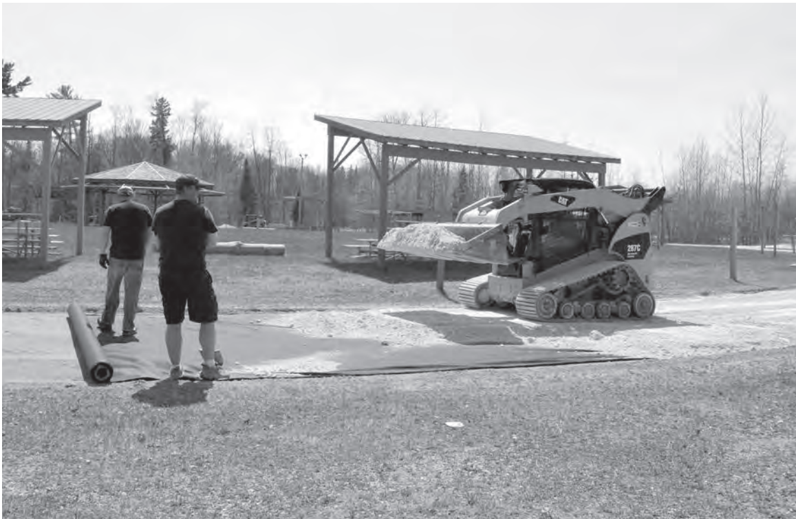
Sault Tribe Construction work crew spreading crushed limestone on the Ring Road around the powwow grounds. Left to right: Joe Paquin, Mike Romano and operating the Skidsteer is Jeff Tamlyn.
