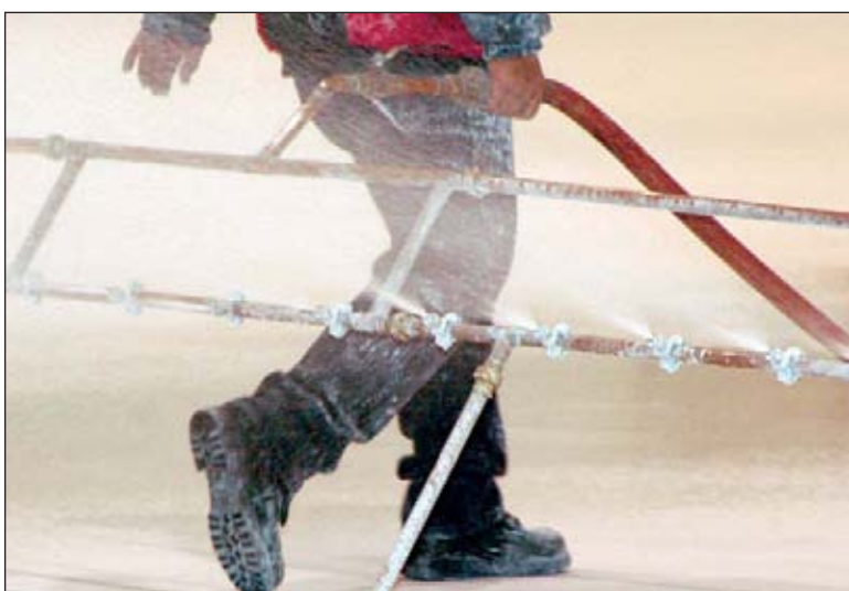
Spray boom putting a seal coat of water on top of the ice.
