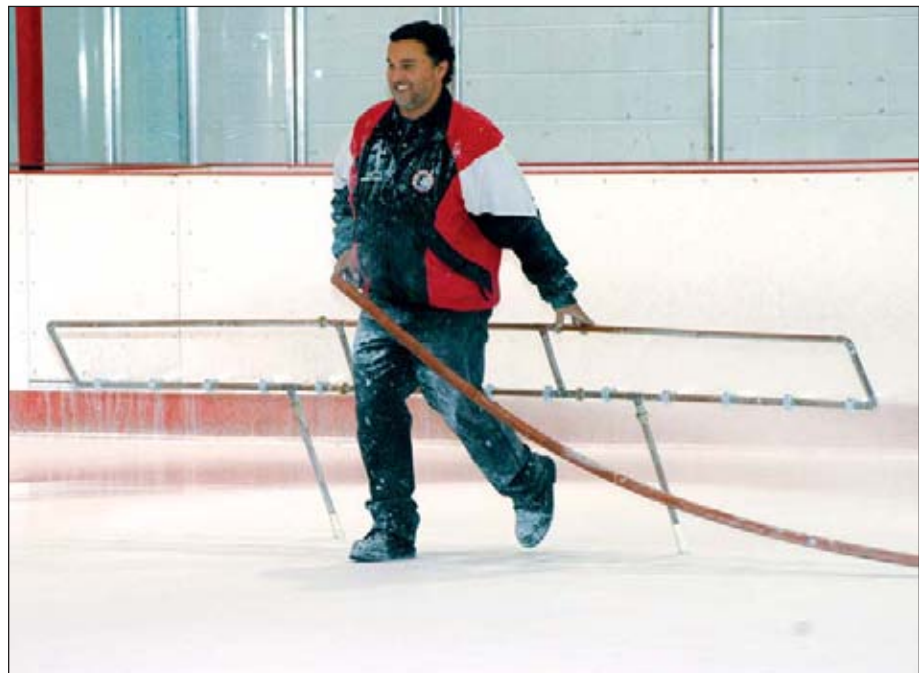
Chi Mukwa Operations Manager Rod Hutte with the spray boom putting a sealant coat of ice on the base layer of white paint.
