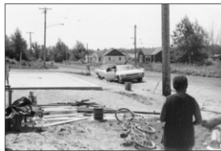
View from Rosemary Gaskin's home. Laurie Gaskin looking at new playground concrete.
