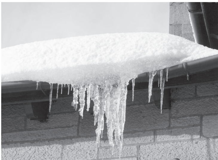
Ice dams like the one photographed above are a sign of a building's heat escaping through the exterior.
