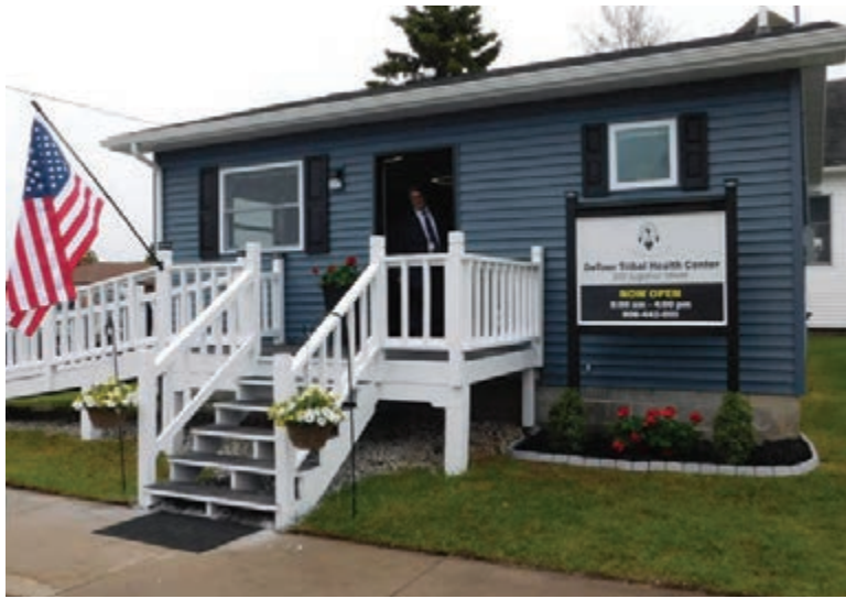
This former beauty salon, located at 200 St. Mary's Street in DeTour Village, has been converted to the DeTour Tribal Health Center which officially opened on May 19.
