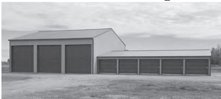
New storage facility at the tribe’s Odenaang Housing site in Sault Ste. Marie. Another recent development in creating sources of revenue.
