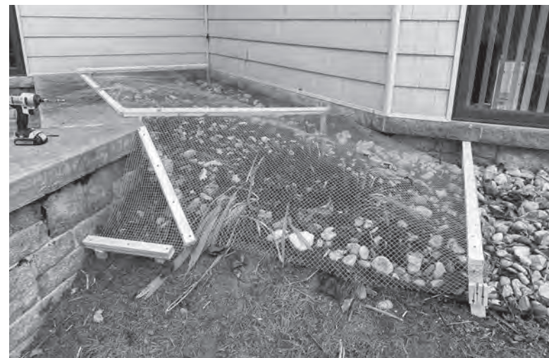
Metal hardware mesh may provide a mechanical method for controlling Japanese knotweed.
