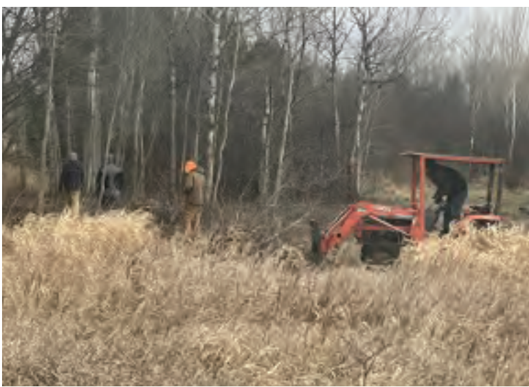
Professional tree removal in progress.
