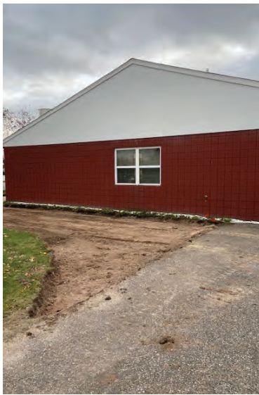
Construction gets underway in preparation for the new window.
