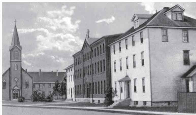
Harbor Springs Holy Childhood of Jesus was opened in 1829. It was closed from 1839 until 1884, when it reopened. The boarding school officially closed in 1983, but continued as a day school, daycare center and thrift shop. It was demolished in November 2007.
