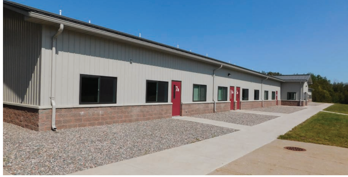
The newly constructed Anne Suggitt Early Childhood Center opened Spring 2021.
