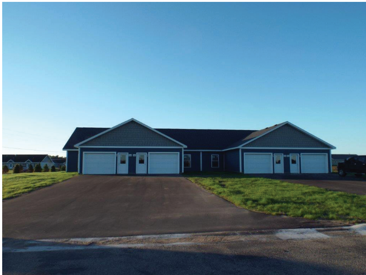
The elder ADA four-plex building four units of two-bedroom units was 90 percent complete at the end of 2021.
