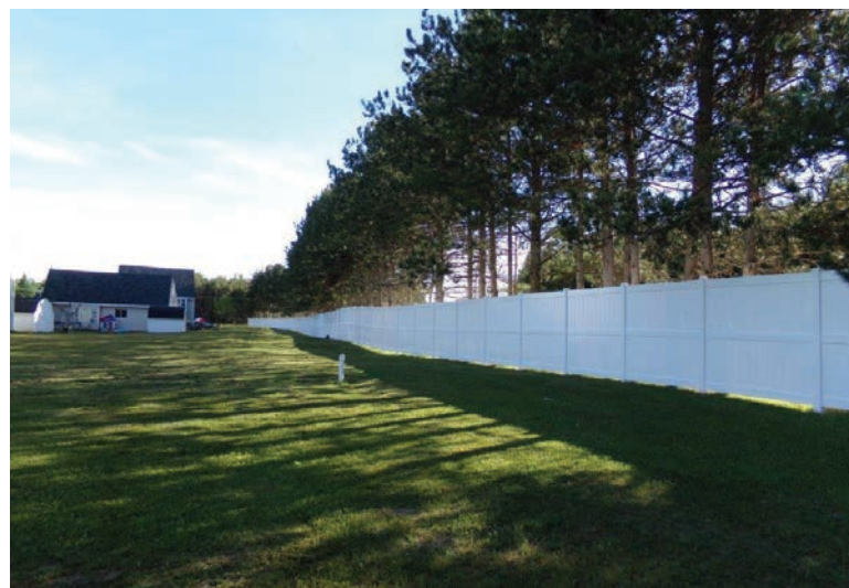
To ensure safety, the Housing Authority placed a 540-foot fence along the edge of the Manistique Housing site.
